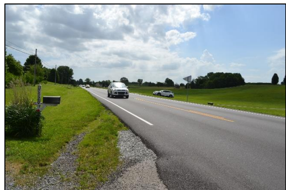
Substandard Shoulder along Corridor 1
